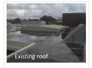
The original bitumen felt roof covering on Cheadle Hulme High School had been refurbished at some point with a liquid applied waterproofing system, but still retained a lot of ponding water after rainfall. This in turn was leading to the growth of algae and moss on the roof surface which created danger for anyone accessing the roof for maintenance.
