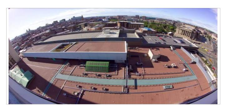
The roof covering at St Johns Shopping centre in Liverpool had seen better days at it had come to the end of its natural life cycle. BBR was the successful roofing contractor engage by the client Land Securities to refurbish and upgrade the existing waterproof system. After liaising with the nominated waterproofing manufacture Tremco, a no heat system was chosen for logistical and financial reasons.
