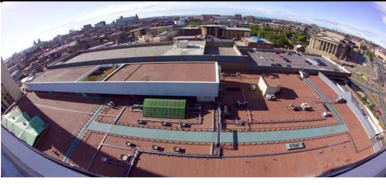
The roof covering at St Johns Shopping centre in Liverpool had seen better days at it had come to the end of its natural life cycle. BBR was the successful roofing contractor engaged by the client Land Securities to refurbish and upgrade the existing waterproof system. After liaising with the nominated waterproofing manufacture Tremco, a no heat system was chosen for logistical and financial reasons.
